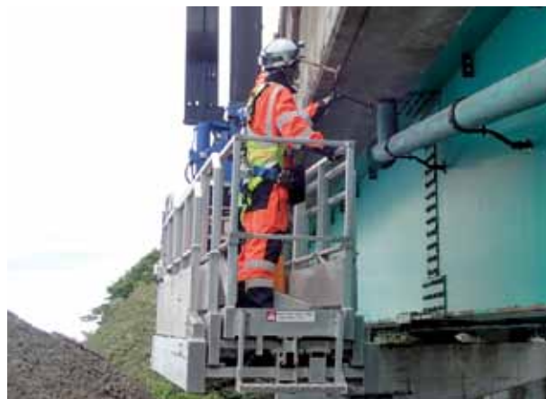
橋梁の打音点検
