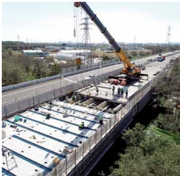
橋梁の床版取替
